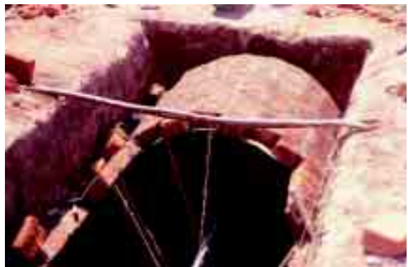
Plate 3.4 Layout and excavation of sausage-shaped tank.
