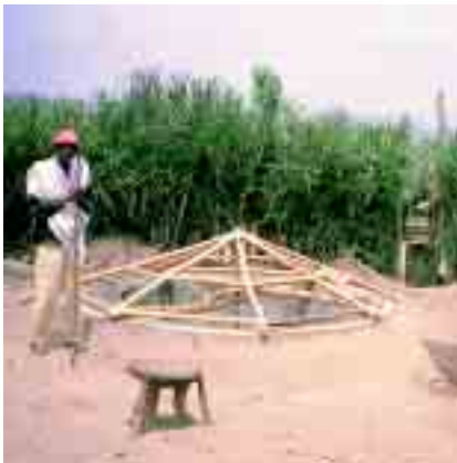
Plate 2.3 Construction of roof.
