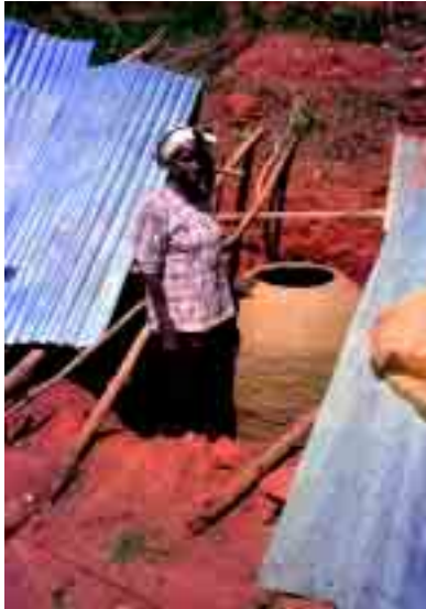
Plate 3.1 Self-standing underground ceramic tank after firing but before back-filling with soil.
