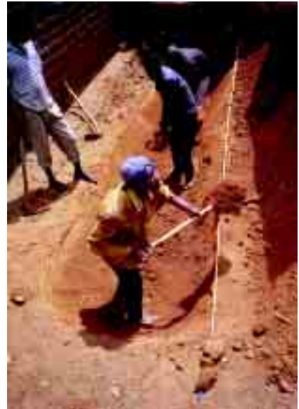
Plate 3.4 Layout and excavation of sausage-shaped tank.
