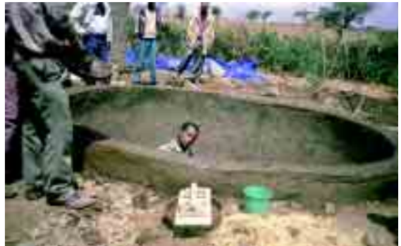
Plate 2.2 Completion of tank lining.
